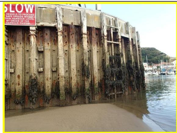
Corroded sheet piling and damaged timber fenders at end of West Pier
