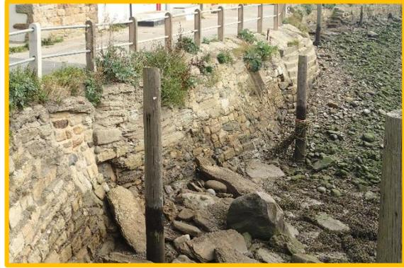
Missing pointing and voids in wall and displacement of toe armour.
