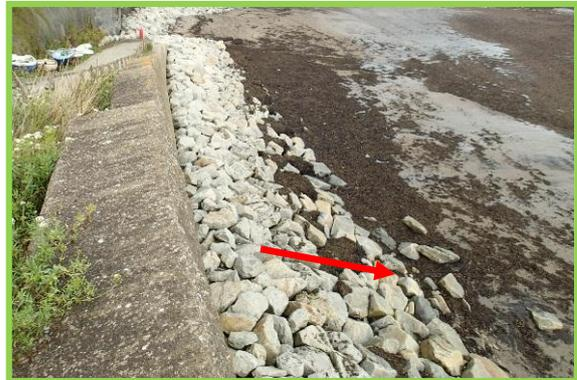
Section of rock armour with gaps / displaced units in front of 2001 seawall. (Asset Ref. 1221D901D1003C01)
