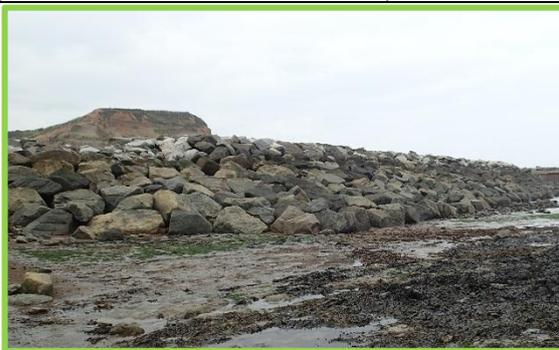
South breakwater outer face rock armour in good
