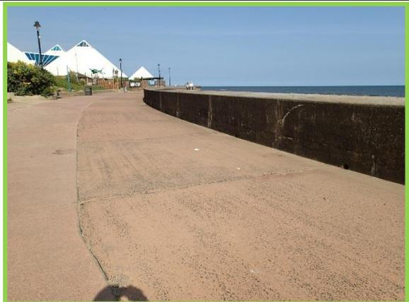
Promenade at Sea Life Centre in good condition. Some cracking to wave wall (Asset Ref. 1221D901D1201C02)
