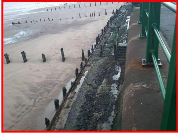
Failed timber groynes and timber breastwork at toe of wall in front of Sandsend **photo from 2012**
