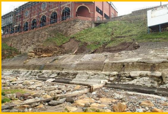
Concrete revetment toe in poor condition and slumps and failures in cliff below building.
