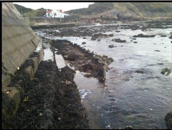
Exposed toe at Sea Life Centre. Note missing infill apron behind end of sheet pile toe. **Photo from 2012** (Asset Ref. 1221D901D1201C02)
