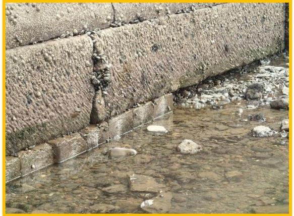
Exposed timber foundation under inner face of east breakwater **photo from 25/09/2014.**
