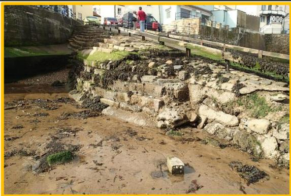
Damaged and missing blockwork to slipway (Asset Ref. 1221D901D0403C05)
