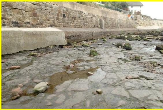
Exposed mudstone platform and undermining of wall toe 12/09/2014
