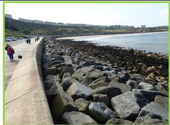
View of crest wall and rock armour with toe piles
