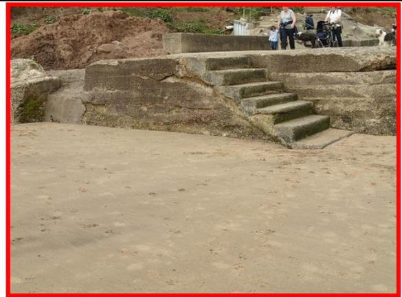
Repairs have been undertaken to patch up the defence at beach access south of the pumping station. (Asset Ref. 1221D901D1402C06)
