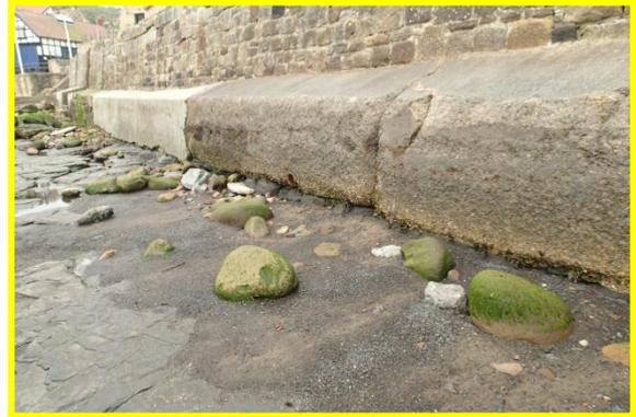
Undermining of wall toe 12/09/2014
