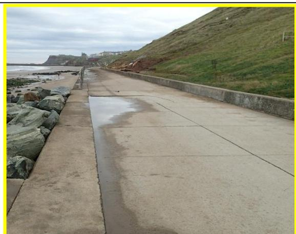
Promenade looking south east showing cracks in slabs and standing water **Photo from 2014, (compare to 2012 photo left)** (Asset Ref. 1221D901D0801C01)
