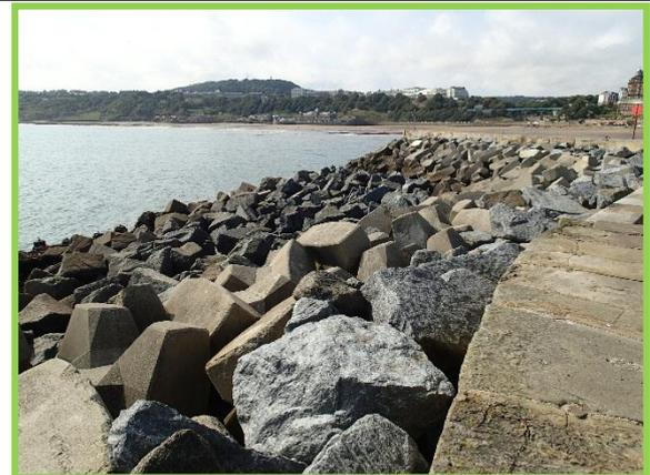
Tightly packed rock armour, Accropodes rock toe blanket and concrete toe piles seaward of East Pier harbour wall
