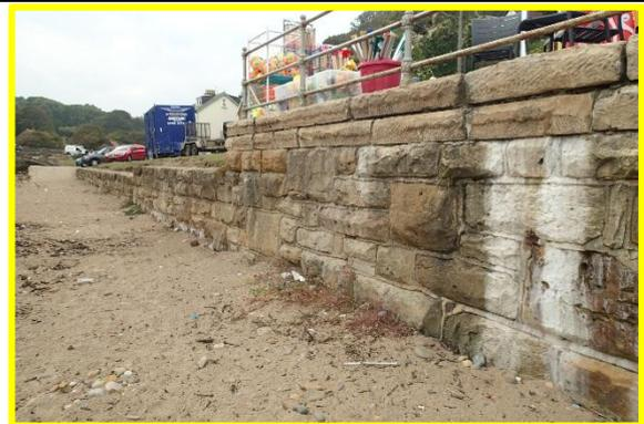
Low masonry wall at east Row Beck, north bank. Damage including missing blocks and mortar adjacent to beach shop. (Asset Ref. 1221D901D0702C03)
