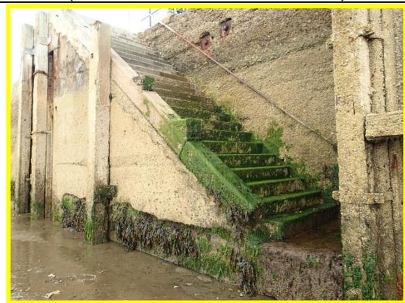
Cracks to concrete facing and exposed toe to steps on West Pier
