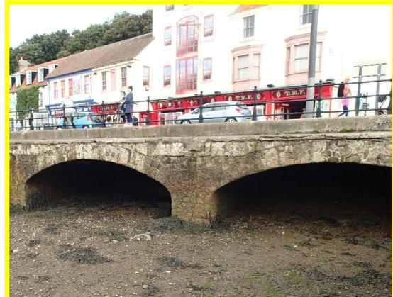
Spalling concrete capping to arched suspended quay at east end of Sandside
