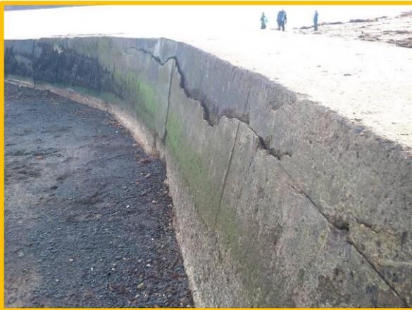
Large horizontal crack to breakwater photo from 2012. (Asset Ref. 1221D901D0601C02)
