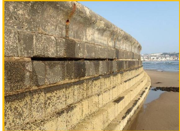
Repaired upper section of upper wall adjacent to re-constructed concrete ramp. (Asset Ref. 1221D901D1303C02)
