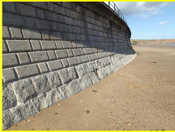
View of wall looking north from near Crescent Hill access, showing abraded lower facing blocks. (Asset Ref. 1221D901D1602C03)
