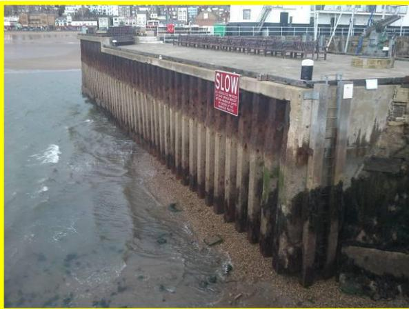
Corroded sheet piles, but overall fair condition
