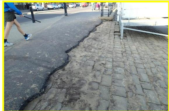
Damage at edge of road and open joints in some of the beach access ramp blockwork. (Asset Ref. 1221D901D1301C23)
