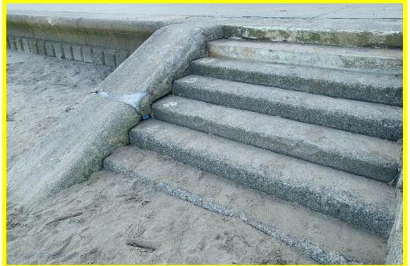
Abrasion damage rounding steps and washout of joints. Asset Ref. 1221D901D1201C17
