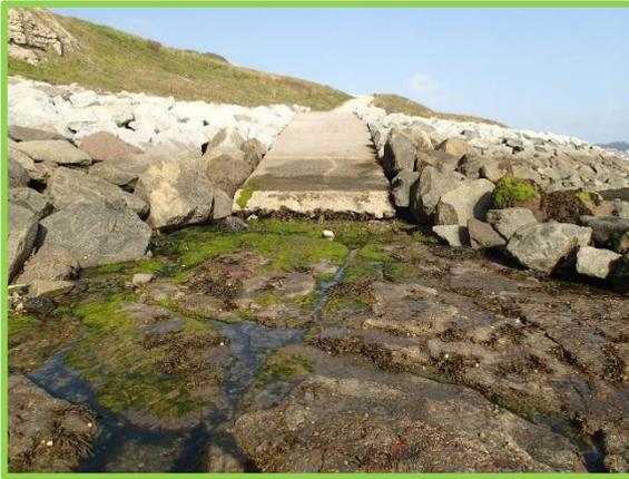
Vertical drop off ramp at south end of Holbeck revetment (Asset Ref. 1221D901D1304C01)
