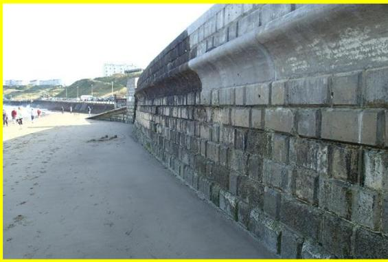
Damage to lower blocks on southern section of wall at Peasholm Gap.
