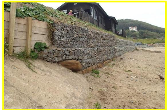
New section of gabions protecting café at NW end of revetment, **12/09/2014**. (Asset Ref. 1221D901D0702C02)
