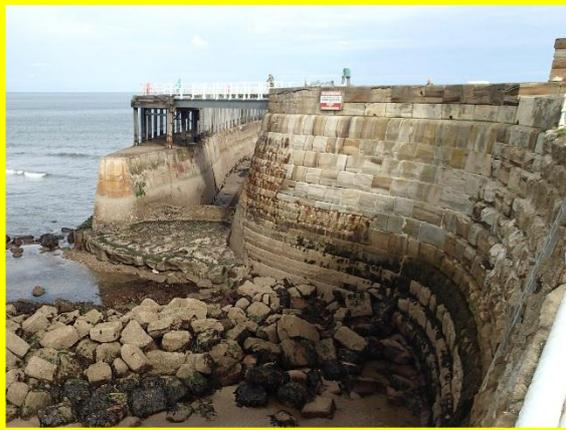
Undermining of apron between main and outer West Breakwater (Asset Ref. 1221D901D0803C02 / 01)
