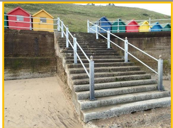
No change from 2009 to stair sidewalls, but new handrails. (Asset Ref. 1221D901D0802C04)
