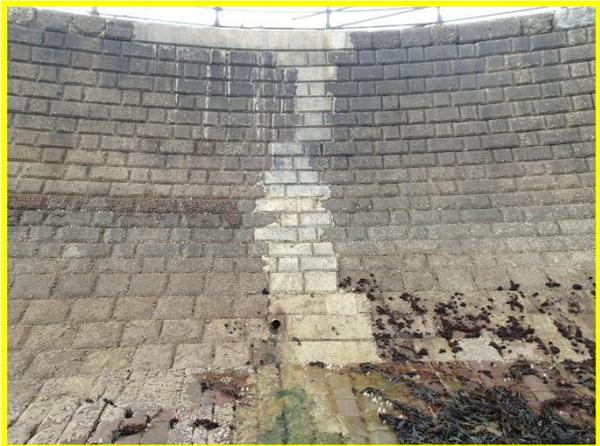
Repair to vertical crack and capping beam north of the ramp. (Asset Ref. 1221D901D1201C21)
