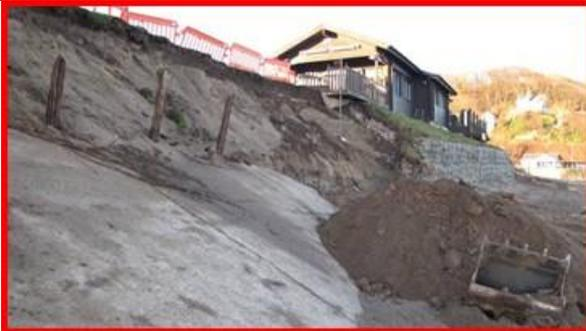
Corner of gabions protecting café at NW end of revetment being repaired, **17th December 2013**. (Asset Ref. 1221D901D0702C02)
