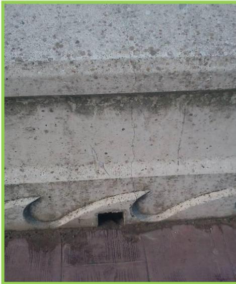
Example of crack through centre of wave wall –
