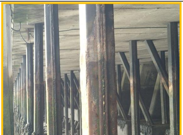
Corrosion to deck support columns
