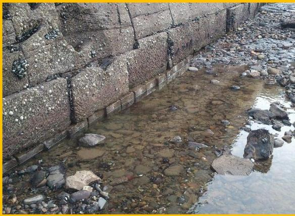
Exposed timber foundation under inner face of east breakwater **photo from 2012.**
