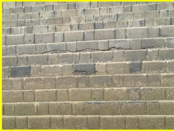
Horizontal cracking in original blocks
