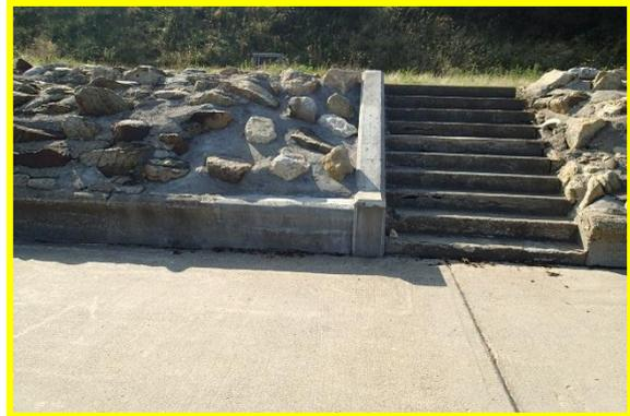
Grouted revetment behind prom has been repaired in many locations Asset Refs. 1221D901D1201C25 & C04
