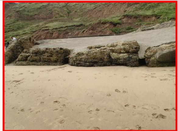
Around 300m south there is a beach access point for the path from the public car park at the surf shop. There are a set of beach access steps that were previously protected by gabion baskets, which have distorted and split under wave action and / or cliff movement, see below left and right. This is not a formal coastal defence, so has no asset number.
