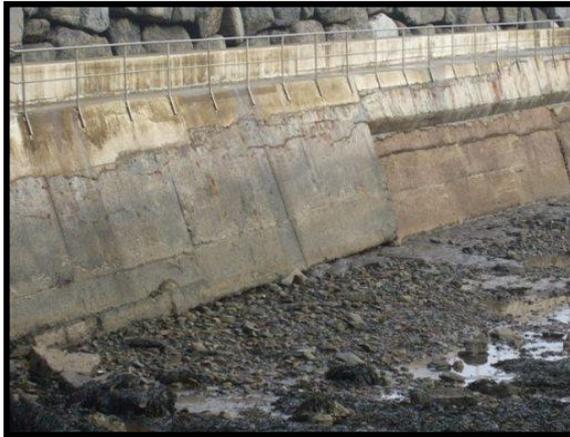
Undercutting to landward facing of north breakwater (photo from 2009 inspection)
