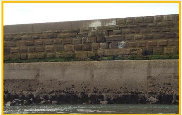
Example area of displaced blocks on outer (W) face of East Pier
