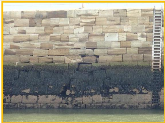
Area of displaced blocks and voids on inner (W) face of East Pier
