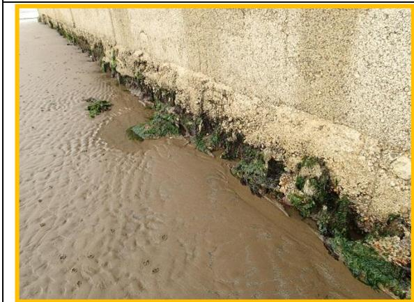
Undermining of toe of concrete encased section at bend where West Pier narrows
