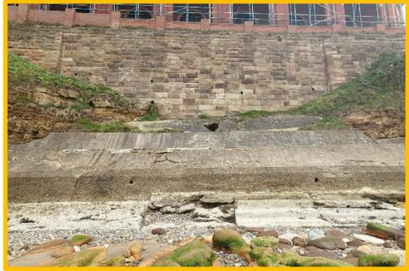
Damage to toe protection and weathering of natural rock below upper wall
