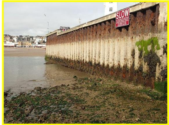
Corroded sheet piles, but overall fair condition
