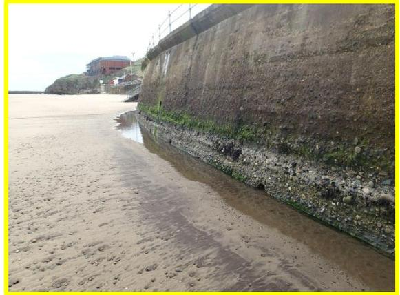
Abrasion damage to wall (Asset ref. 1221D901D0802C14)
