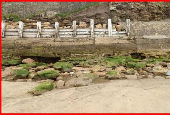
Defence toe undermined with large voids (very poor condition)
