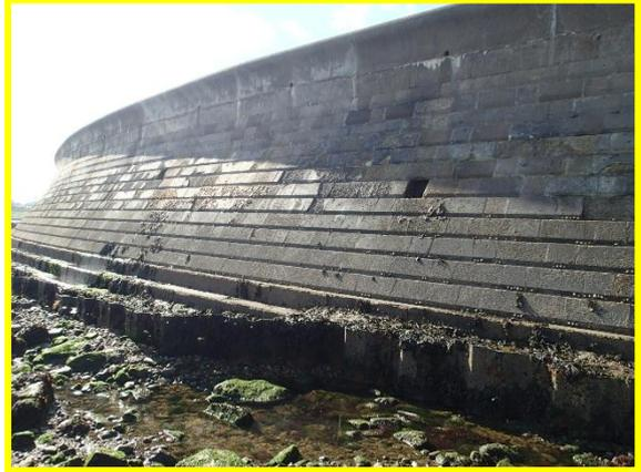
Damage to face of blocks on wall at Sea Life Centre (Asset Ref. 1221D901D1201C02)
