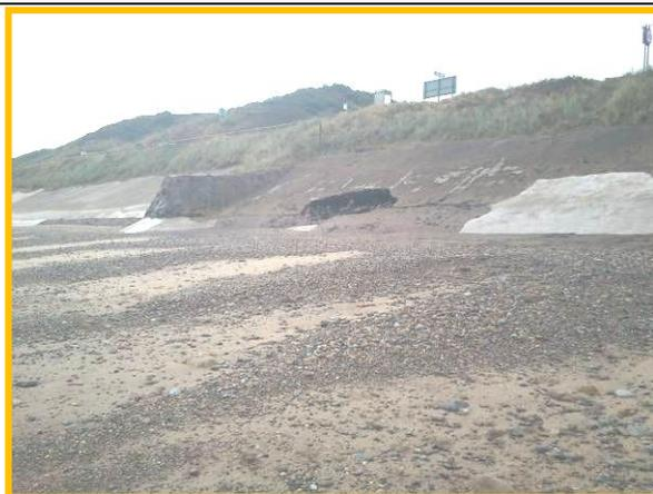
Large void in revetment adjacent to recent patch repair (Asset Ref. 1221D901D0702C02)
