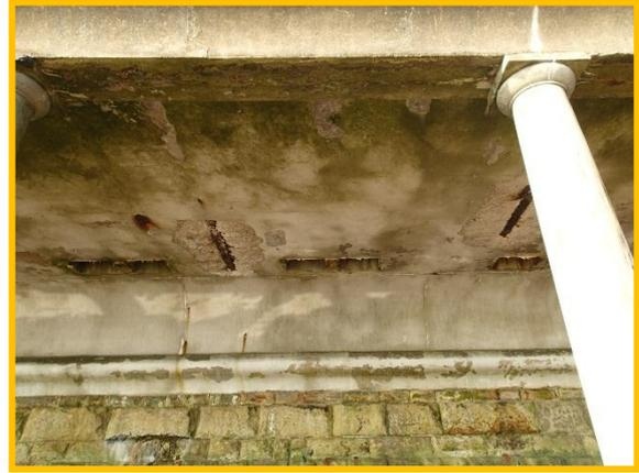
Cracking and corrosion to beams and upper level deck slab (Asset Ref. 1221D901D1302C01)
