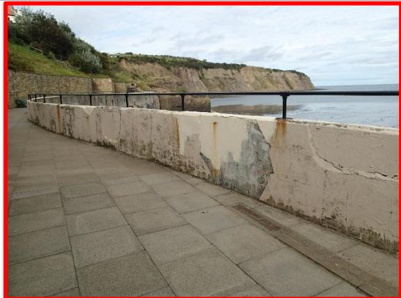
Crest wall locally very poor condition, with evidence of recent cosmetic repairs. (Asset Ref. 1221D901D1003C02)
