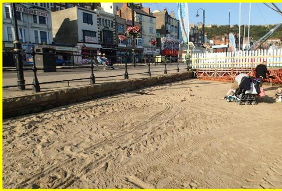
High level beach with only top course of masonry visible, missing mortar. (Asset Ref. 1221D901D1301C22)
