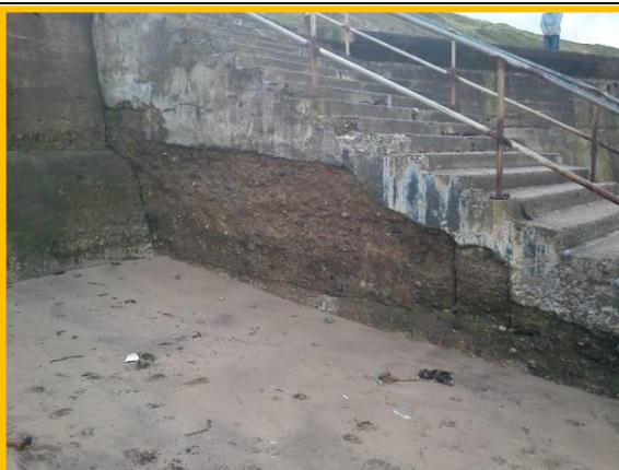
Erosion and cracking to stair side wall - **Photo from 2012** (Asset Ref. 1221D901D0802C04)
