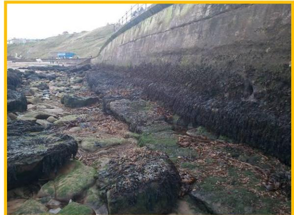
Undermining of toe in section with no rock armour
