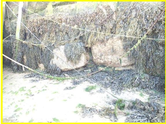
Open joints and voids between blocks in inner face of east Pier below repaired section. (Asset Ref. 1221D901D1301C16)
