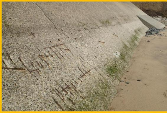
Abrasion damage to revetment exposing reinforcement.
