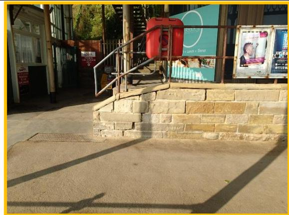
Weathering and loss of joints in stone wall at back of high level prom by cliff railway
