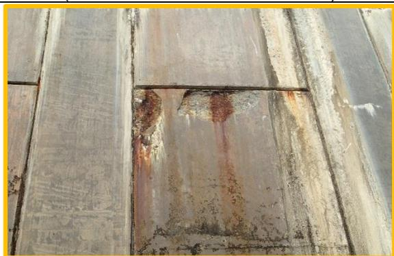
Example of typical damage to precast panels (Asset Ref. 1221D901D1003C02)
