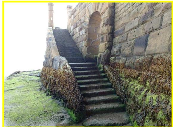
Abraded and slippery steps with rounded edges makes beach access hazardous. (Asset Ref. 1221D901D1301C27)
