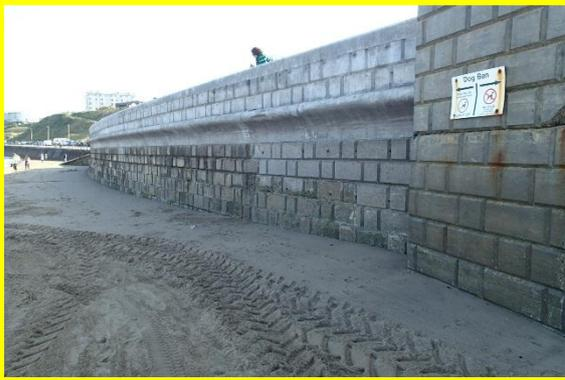
Repaired section of upper wall and splash beam at Peasholm Gap.
