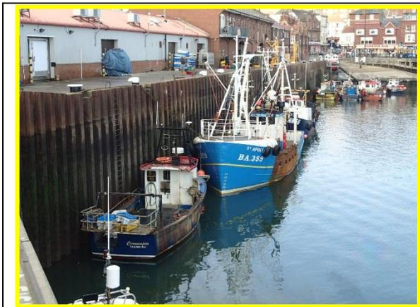
Corroded sheet piling of West Pier
