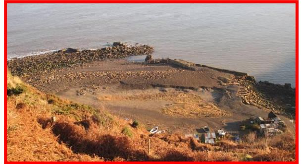
Overview of asset in Dec 2013 following storm surge of 5<sup>th</sup> Dec 2013. Significant loss of fill material adjacent to the breakwaters since July 2013 (left). (Asset Ref. 1221D901D0502C01)
