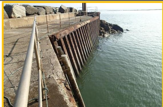
Corrosion of sheet piling on the landward side of the north breakwater (12/09/2014) (Asset Ref. 1221D901D0402C01/4)
