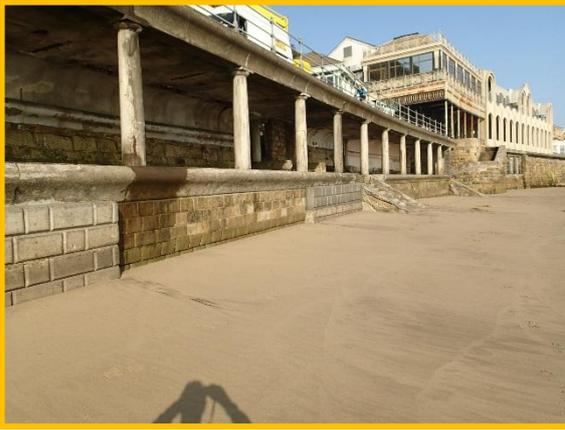
Repairs have been undertaken to lower level wall, but defence remains in poor overall condition (Asset Ref. 1221D901D1302C01)
