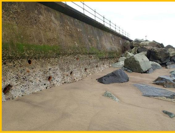
Abrasion damage to lower part of wall
