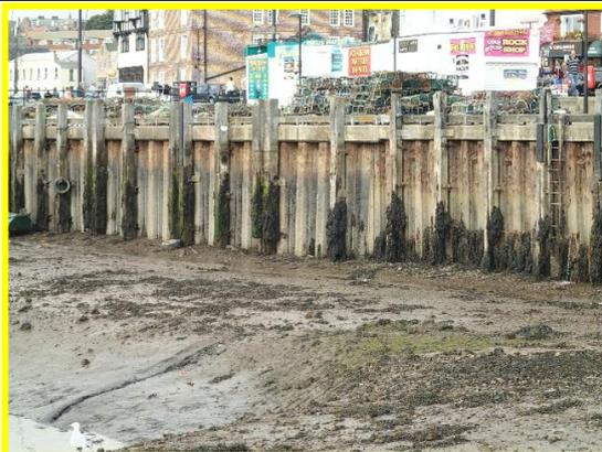
Corroded sheet piles at back of harbour
