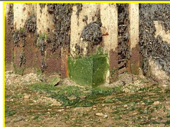
Repair to void under SE corner of breakwater by lighthouse **photo 10/09/2014**
