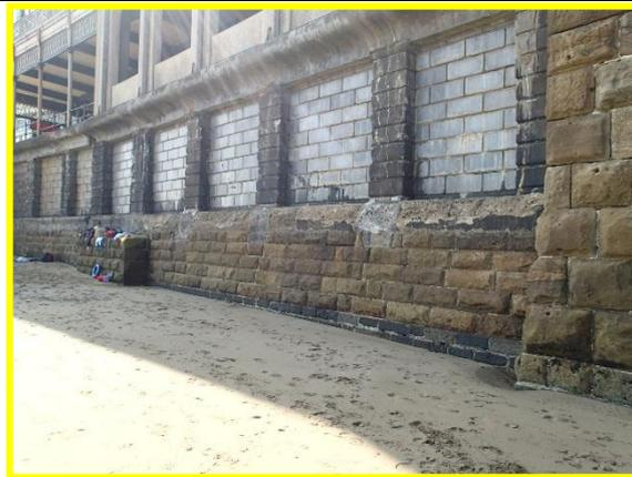
Abraded and spalling concrete capping to original wall below in filled openings
