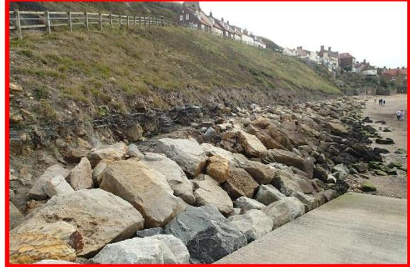
Displaced rock armour and damaged revetment at the Haggerlythe inside harbour adjacent to East pier (Asset Ref. 1221D901D0803C05)
