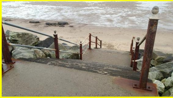
Corroded standards to handrails at steps
