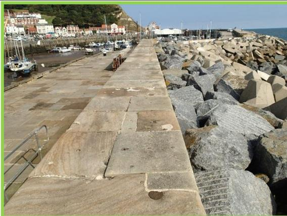
East Pier rock armour and Accropodes showing area of possible settlement of crest armour
