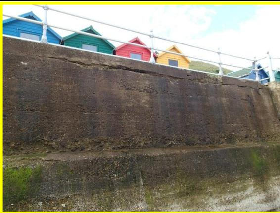
Horizontal cracks in wall (Asset Ref. 1221D901D0802C04)
