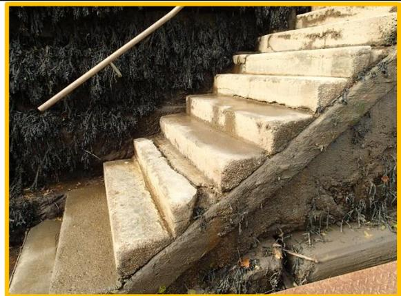
Cracked and loose steps with washed out joints require attention. (Asset Ref. 1221D901D0803C07)
