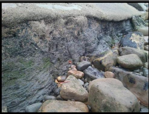
Displaced toe armour, undercutting to concrete revetment and abrasion damage to revetment.
