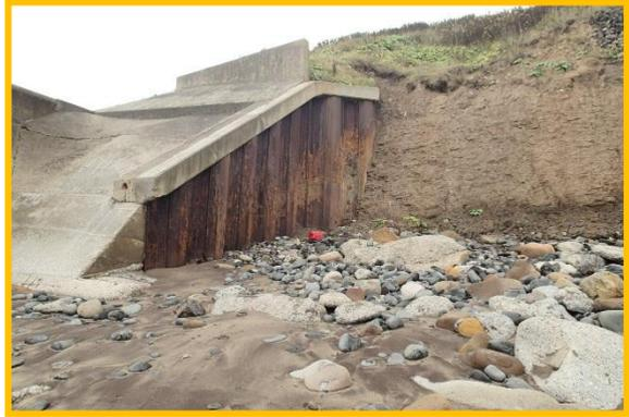
Corroded sheet piling and ongoing erosion at northern end of Sandsend revetment.
