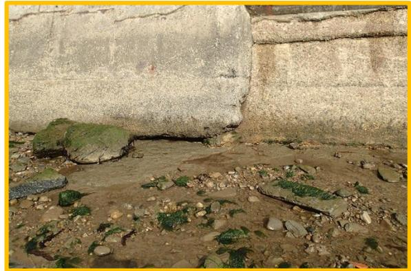
No change since 2009 to undercutting at landward facing of north breakwater (12/09/2014)
