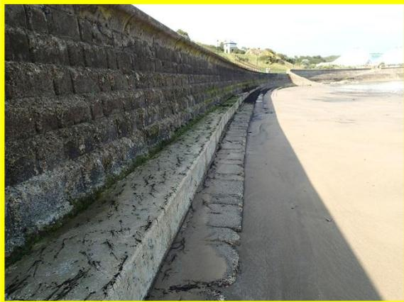
Erosion and spalling of front face of wall. Asset Ref. 1221D901D1201C03
