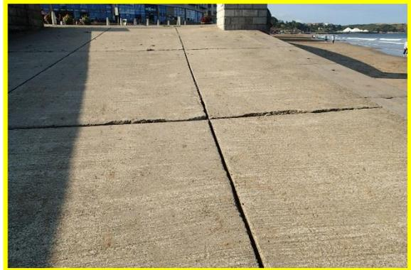
Washed out joints in slipway at Peasholm Gap
